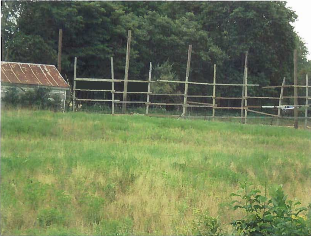
Date: 07/30/2010 Time: 12-1 PM Direction: East Photo by: M. Stevenson Exposure #: 001 Comments: Poles sticking out of the ground.
